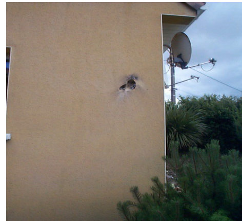
Example 6: Blocks landing in a field and another impact on a dwelling more than 430 m from the blast
