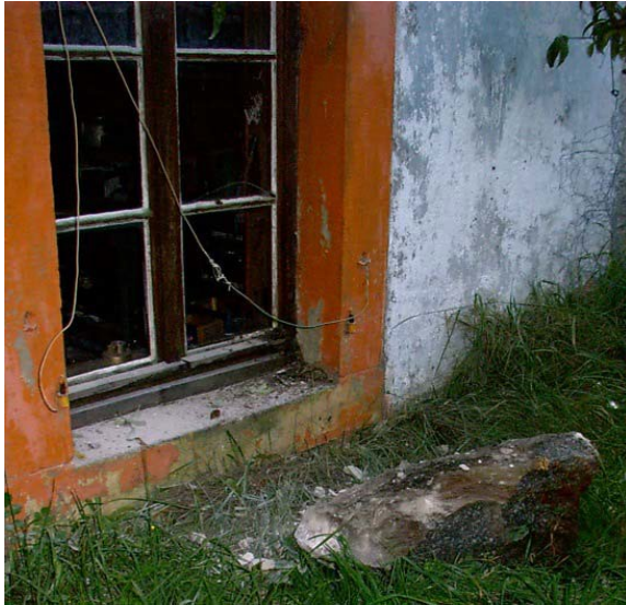
Example 5: Houses bordering a site road and blocks projected onto the frontage approximately 200 m from the blast
