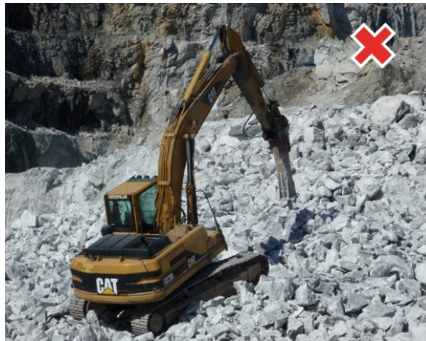
Figure 1: wrong and unsafe oversize hammering treatment.
