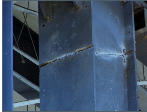
Fig.3 Cut after two Blast attempts
