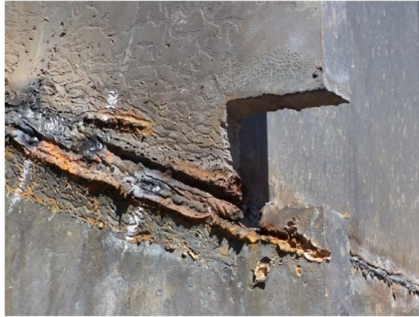
Fig.7 Insufficient Cut After Blast Attempt
