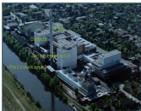
Fig.1 Power Station-View One
