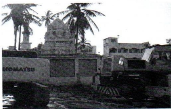
Figure 2 - Sensitive and Critical Structures (Temple and building) at Chikpet Metro Station
