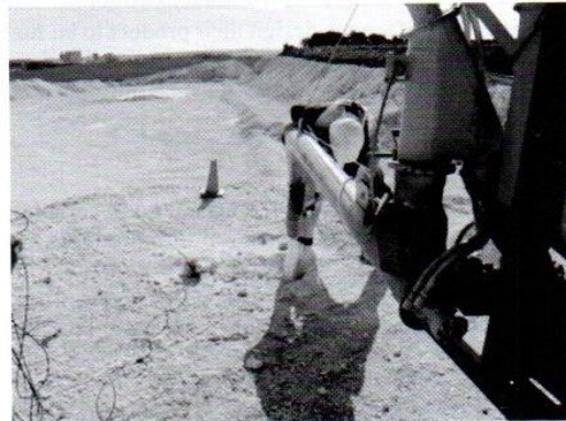
Figure 7 - Charging Blasthole
