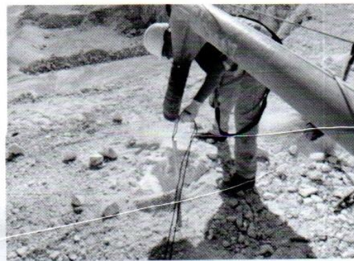
Figure 6 - Loading transducer into a blasthole
