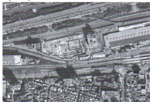
Figure 1(a) - Typical Photograph of the Surroundings near demolition site (shown in red box)
