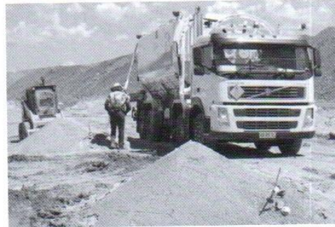
Figure C2 - Final Product being loaded into a Borehole from a Truck
