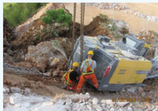
Picture # 3 – Fixing of the drilling machine to the crane
