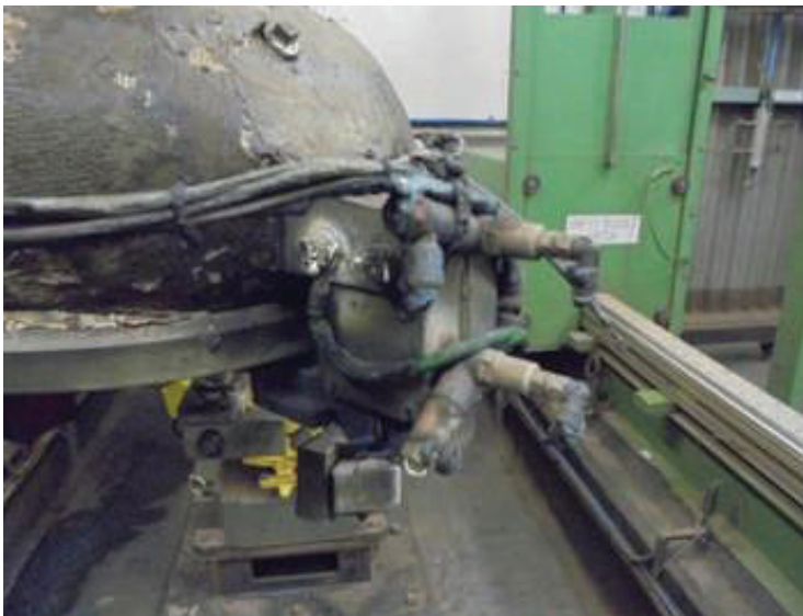
Photo showing damage to the pyrotechnic bucket gripper
