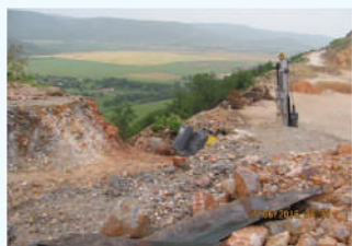
Picture # 7 – Finished road cut
