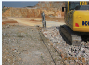
Picture # 4 – Forming of road cut
