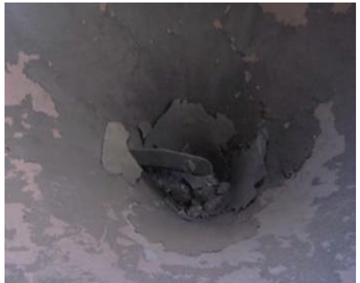
Photo showing inside of drying area vessel with combustion residue
