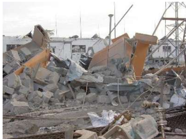
Fig. 2 Explosion in the emulsion plant without separation in Zambia with over 40 fatalities
