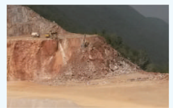
Picture # 14 – Drilling machine after the slide
