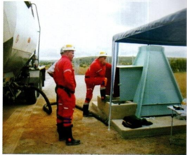
Figure 4 - Transfer in Progress
