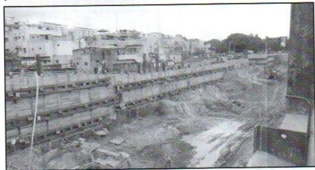
Figure 3 - Blasting Close to Residential Structures at City Railway Station
