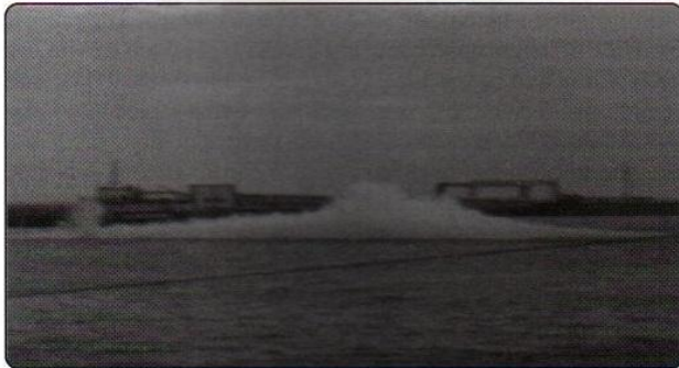
Figure 10 - Underwater Blasting in Progress
