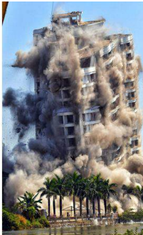
Figure 10: Demolition of Alfa Serene
