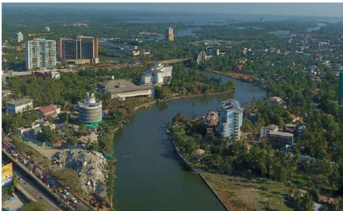
Figure 14: Maradu Apartments after Implosion
