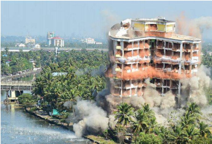
Figure 9: Demolition of Golden Kayalaran
