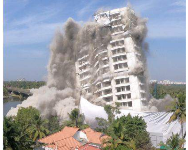
Figure 11: Demolition of H2O Holy Faith
