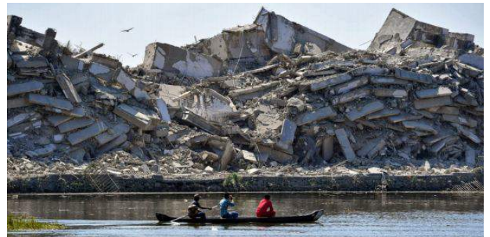
Figure 13: Debris piled after demolition of Alfa Serene
