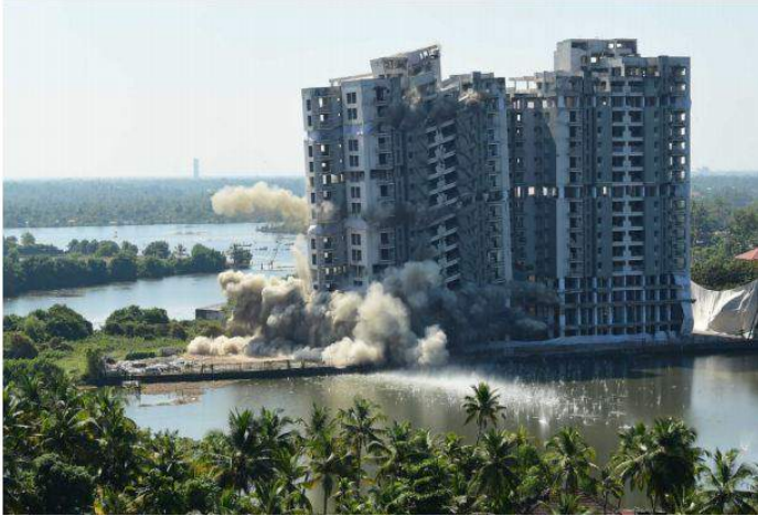
Figure 8: Demolition of Jain Coral Cove
